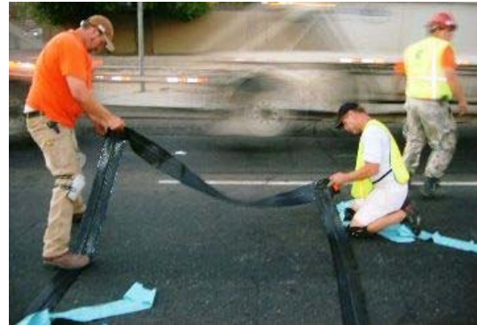
1. Laying Out EzyLoops – Peel and Stick
