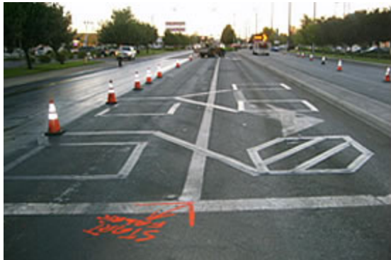
2. EzyLoops Ready for Paving
