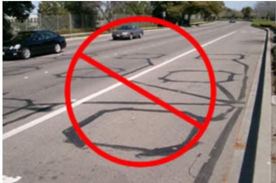
No More Saw-Cuts
